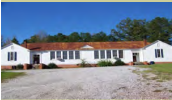
Woodworking Education Center 10544 Hwy 17, Maylene, AL 35114
